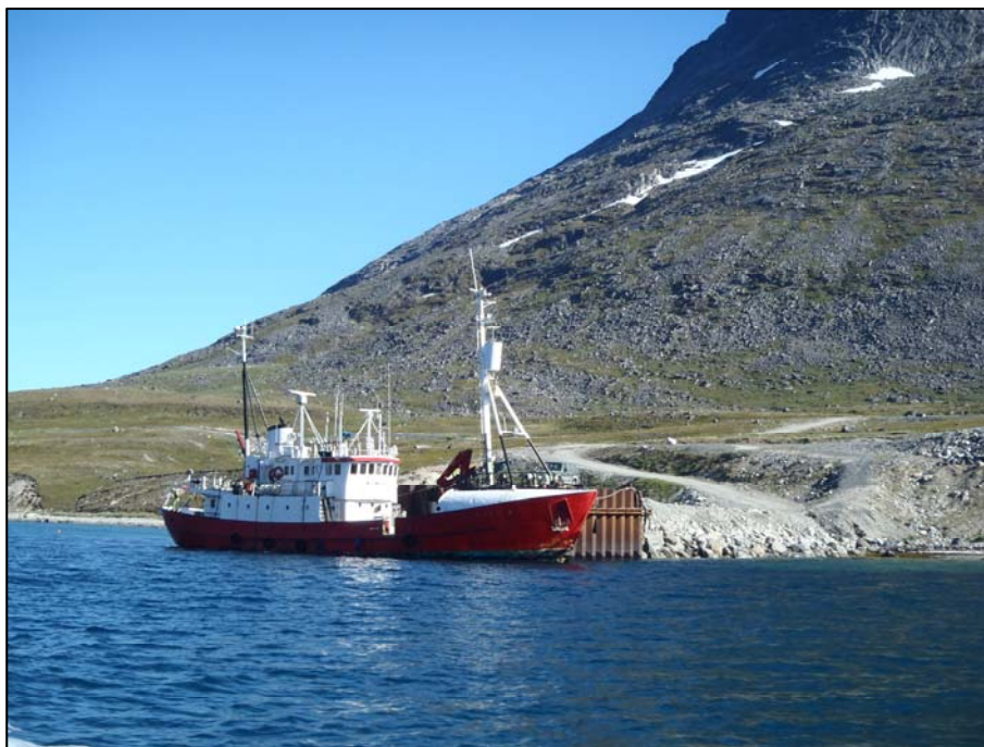
Figure 17-3 The existing quay at Nalunaq harbour, photographed in late June 2016 (source: SRK ES, 2016)
