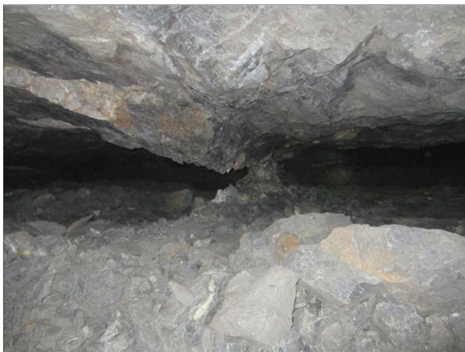
Figure 23-2 Severe pillar damage, pillar loss and excessively wide spans below stope 510-24 resulting from pillar mining. The remaining rock material is not capable of holding any additional hanging wall load (source: SRK ES, 2016)
