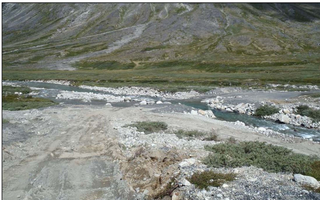
Figure 17-2 Former bridge location over the Kirkespir River where a new bridge will be required. Photographed in in late June 2016 (source: SRK ES, 2016)
