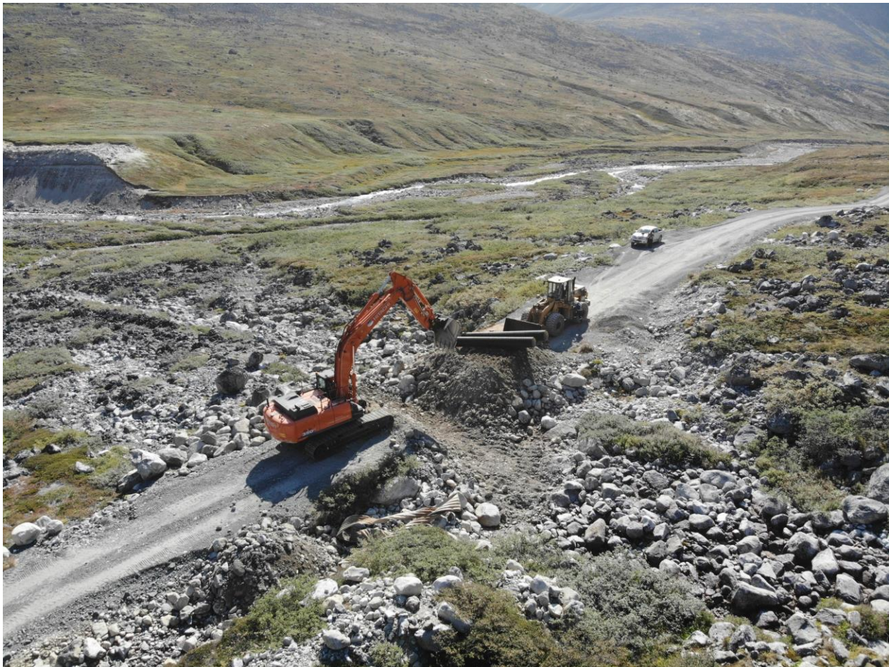
Figure 2: Installation of additional culverts on the mine access road
