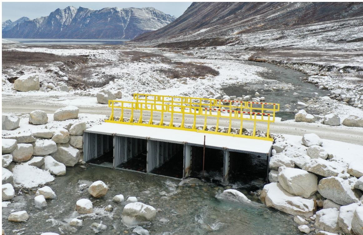
New re-enforced all weather bridge crossing Kirkespir River
