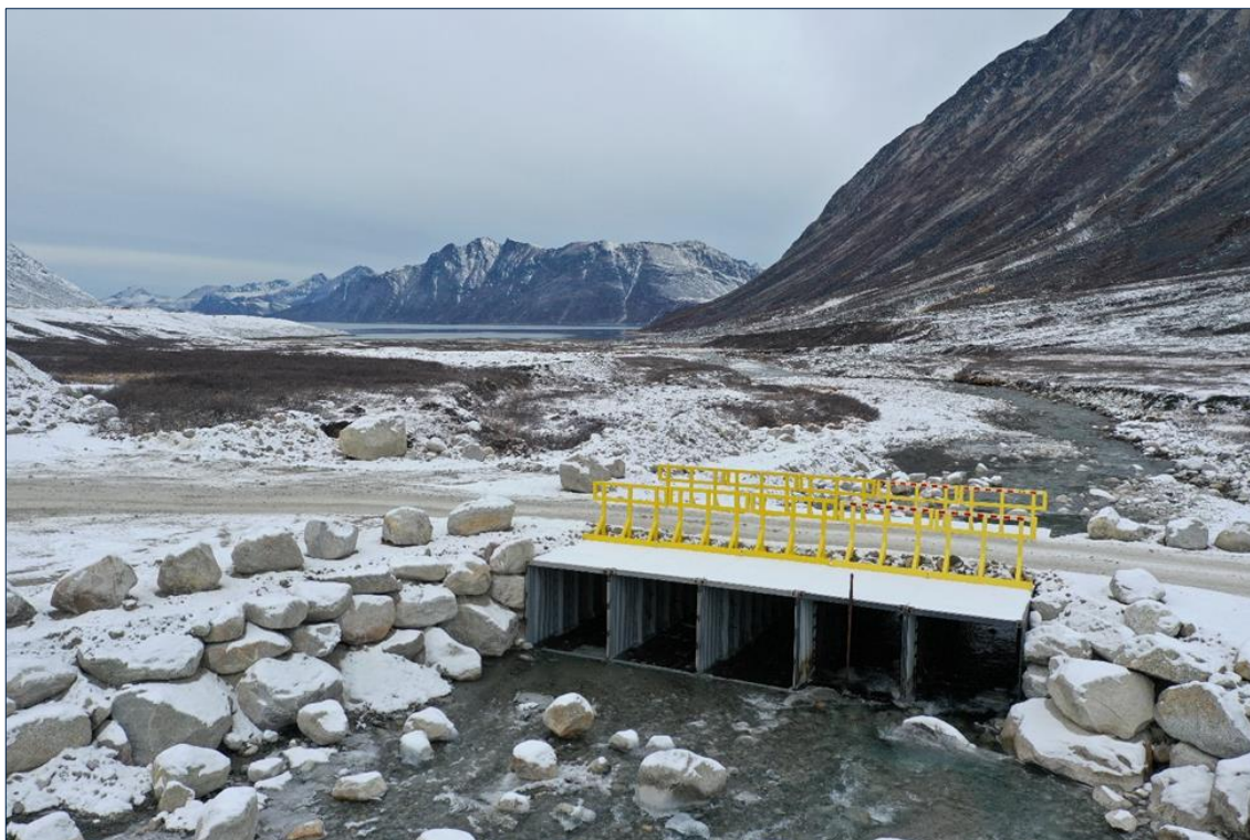
Figure 17-4: Nalunaq - River Crossing bridge structure on site road (Source: Halyard, 2021)
