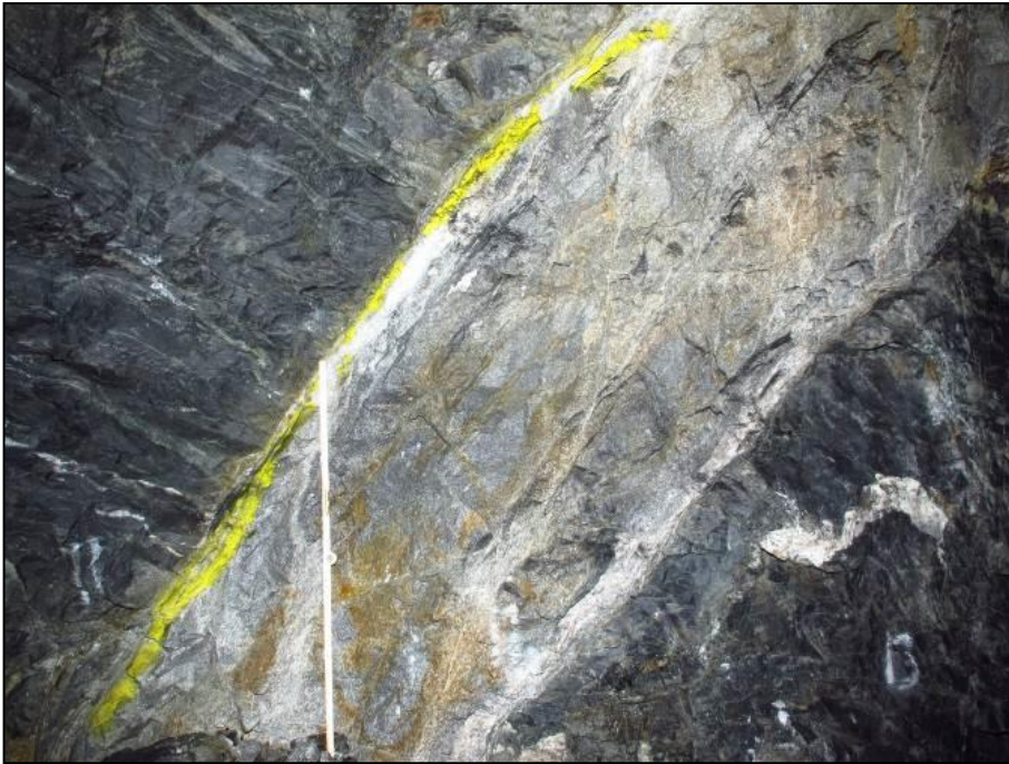
Figure 6-17: Aplite dyke exposed on the wall of the 350 Level West. There is fault gouge at the margins of the dyke indicating movement post-emplacment (Image Source: SRK ES, 2016)
