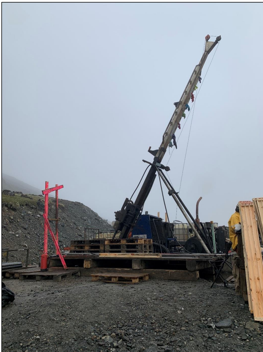
Figure 9-2: Drilling from the prepared pads in 2021
