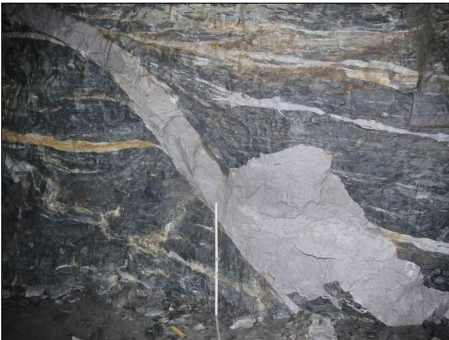
Figure 6-18: Aplite dyke diluting the MV structure on the 600 Level West (Image Source: SRK ES, 2016)
