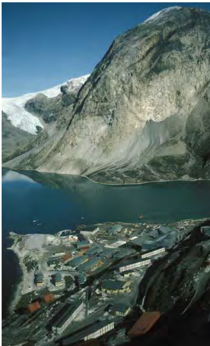
Figure 5-8: View of surface facilities at Maarmorilik and the Angel mountain, summer 1985
