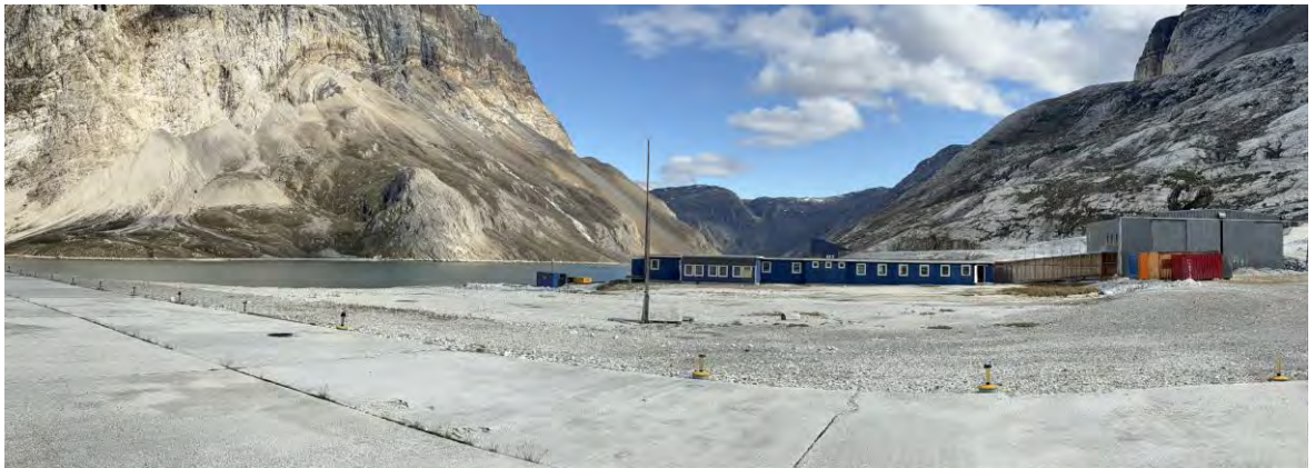
Figure 5-4: Accommodation/offices and warehouse at Maarmorilik, summer 2025
