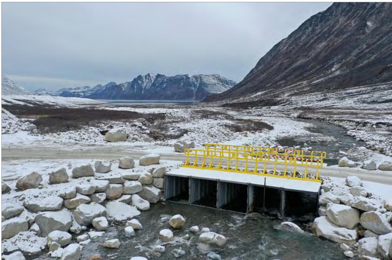
Figure 8-2 River crossing bridge structure, looking southwest
