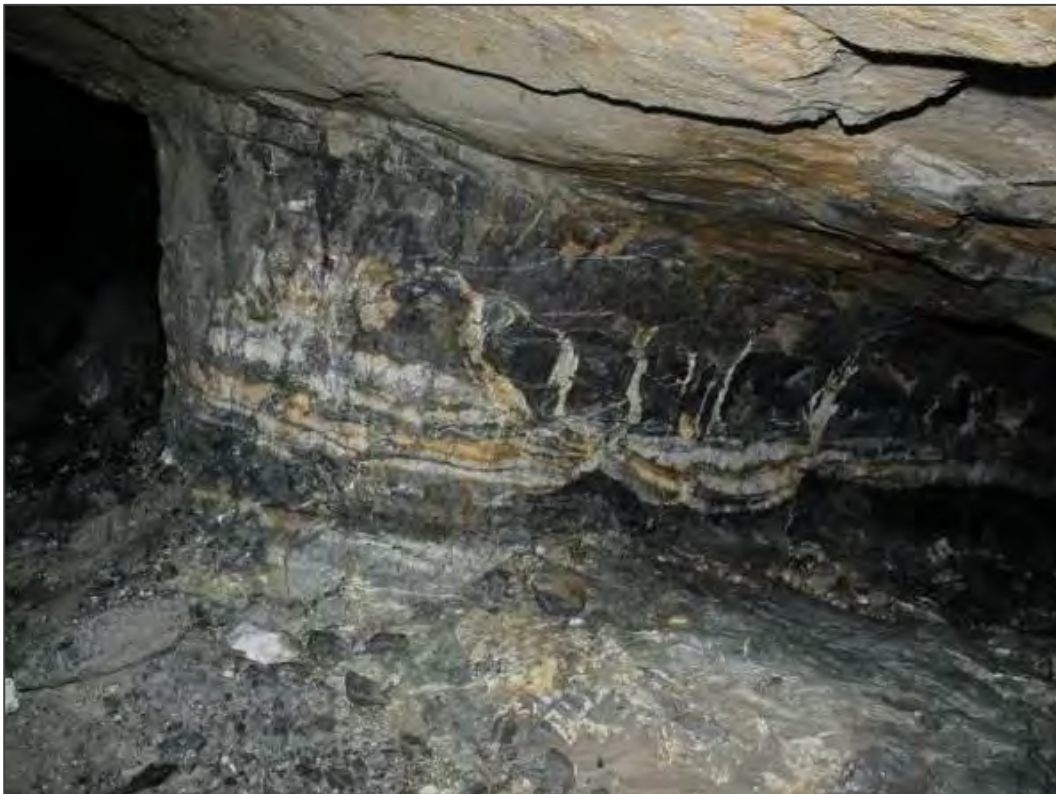
Figure 3-12 Main Vein structure in the Target Block exhibiting quartz-filled tension gashes perpendicular to the vein, indicating brittle deformation
