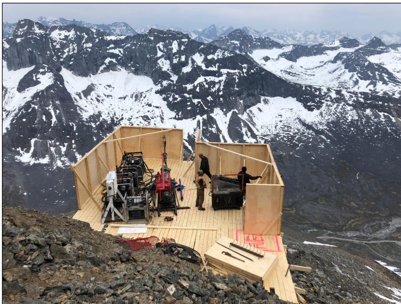
Figure 10-5 Upper drilling platform under construction by IPR in 2023
