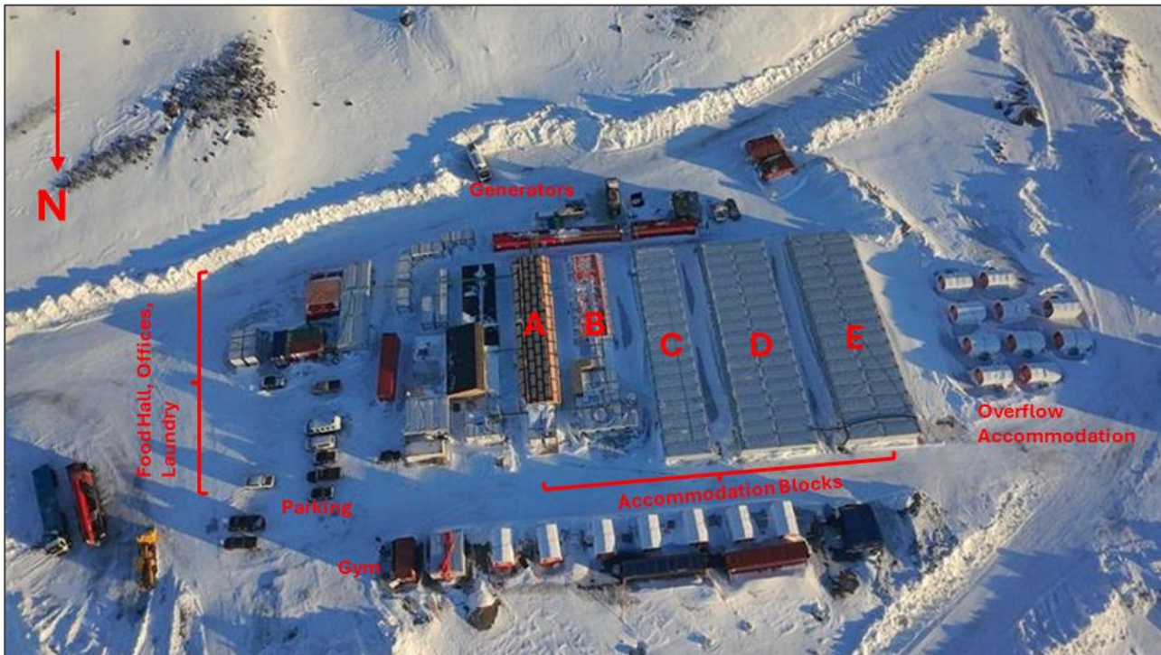
Figure 18-1 Aerial picture of the Nalunaq accommodation camp (accommodation block labelled alphabetically)
