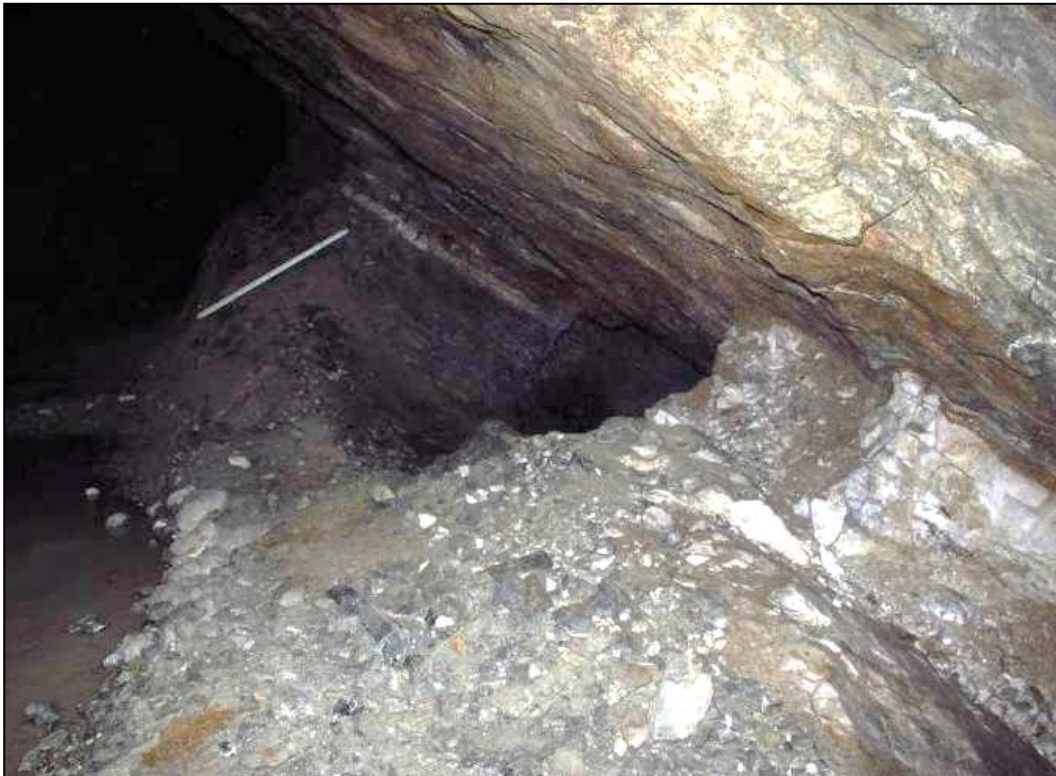
Figure 7-25 Main Vein reducing in thickness from 110 cm in the foreground to 15 cm over a distance of only 4 m in the 390 Level East reef drive
