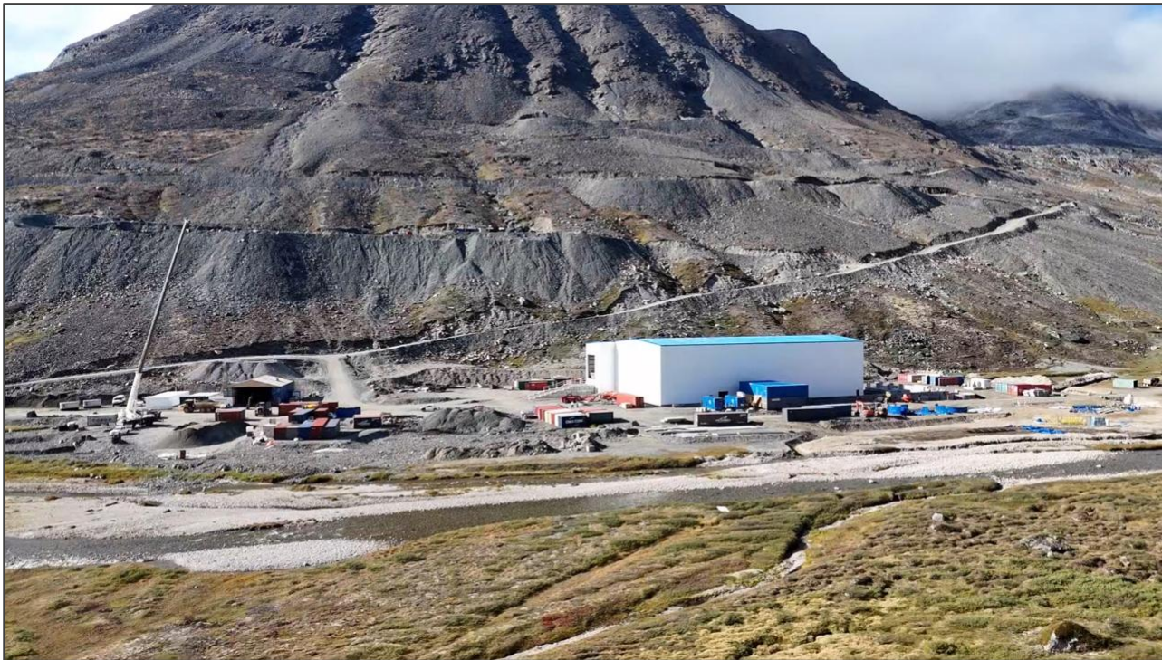
Figure 18-2 Image of the processing facility looking to the west, with Nalunaq Mountain in the background
