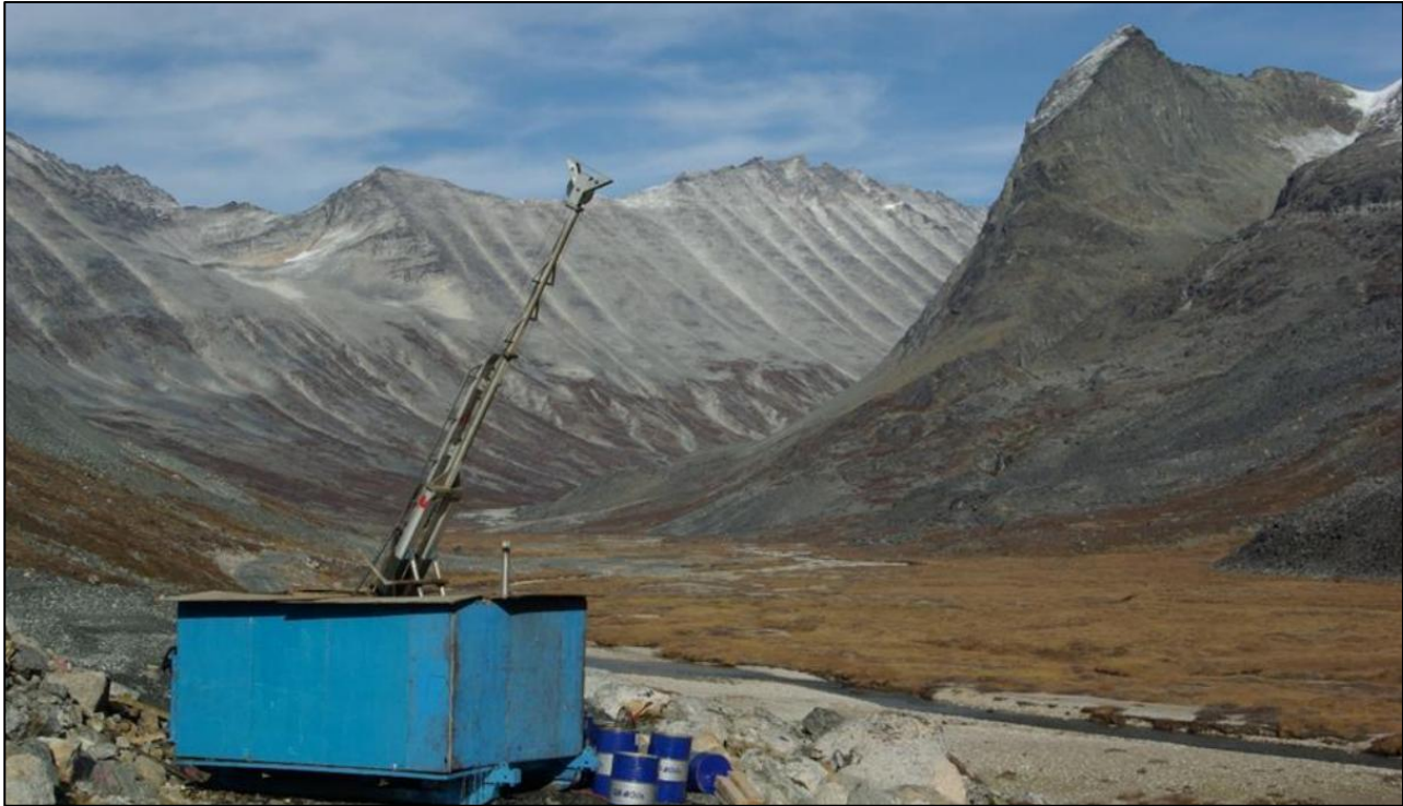
Figure 10-2 Skid-mounted rig drilling from the Nalunaq mine road in 2017
